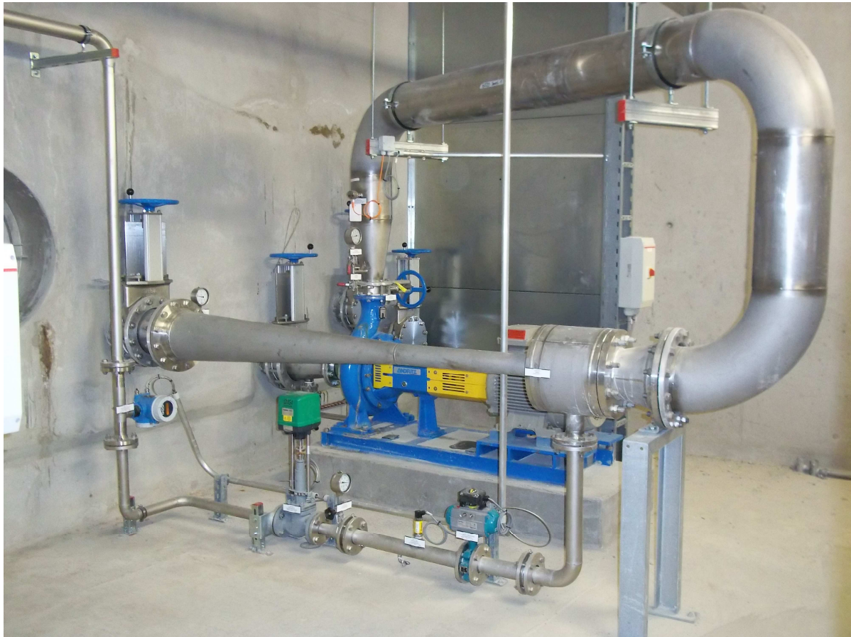
Figure 14: ozone injection and motive water pumps ozone reactor two AOP
