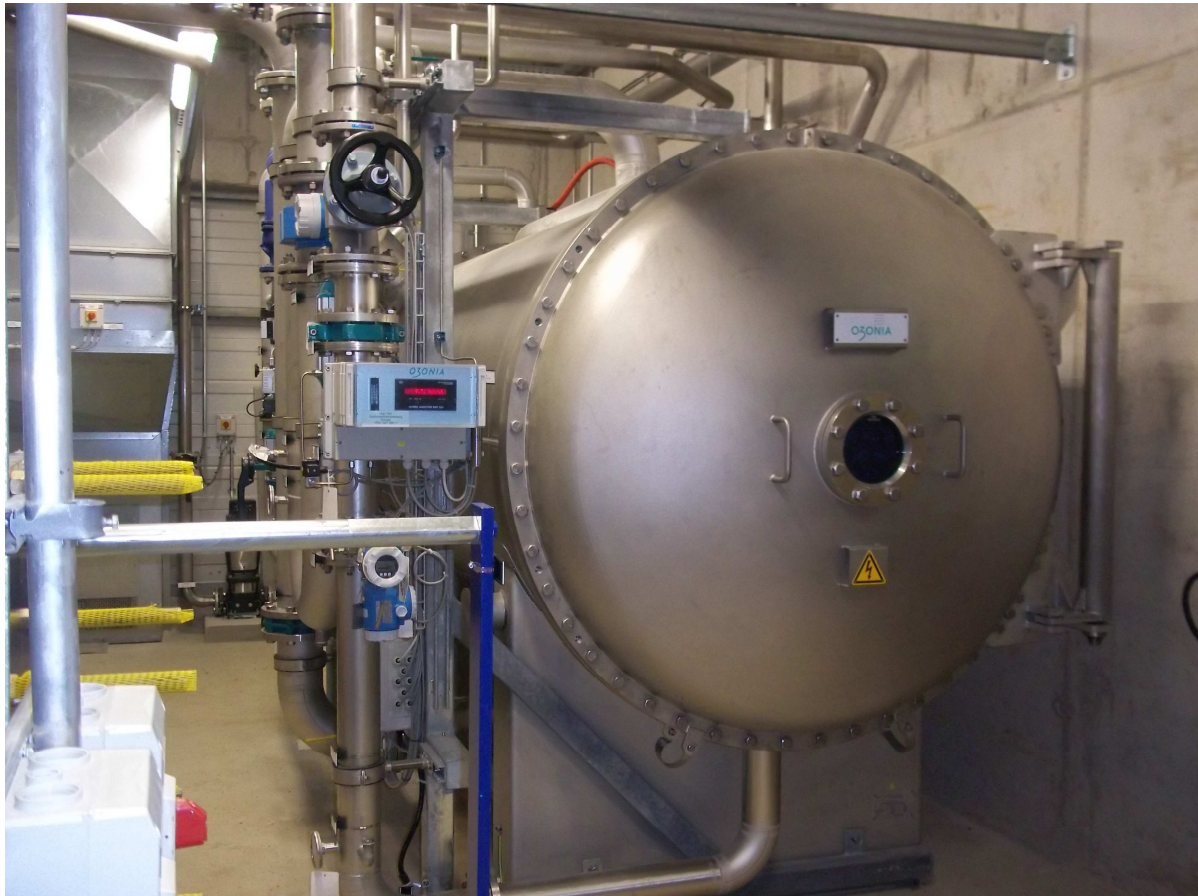
Figure 11: ozone generator AOP
