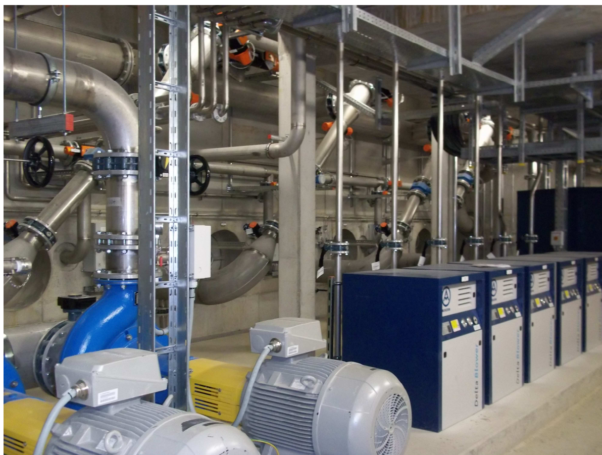
Figure 17: Filter gallery biofilter AOP
