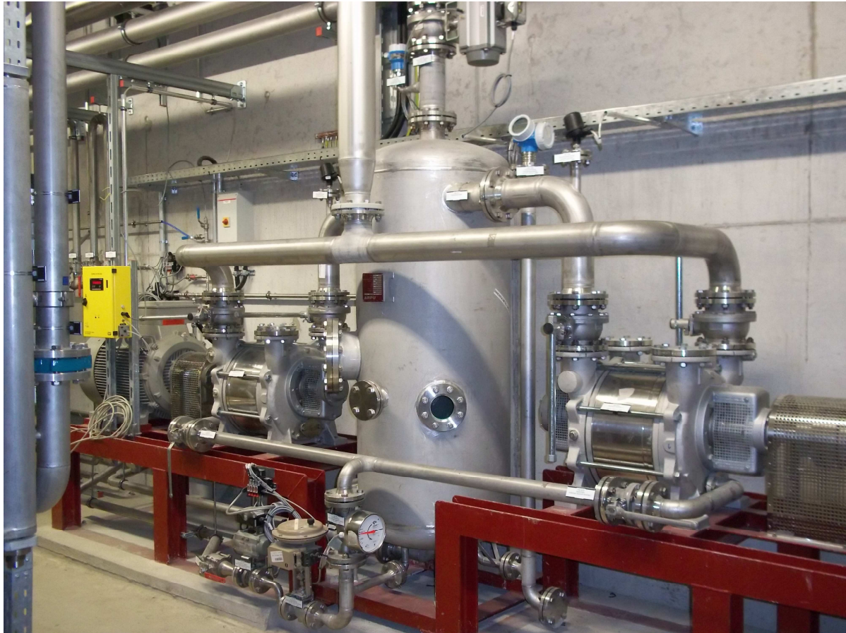
Figure 15: Ozone reactor offgas compressor
