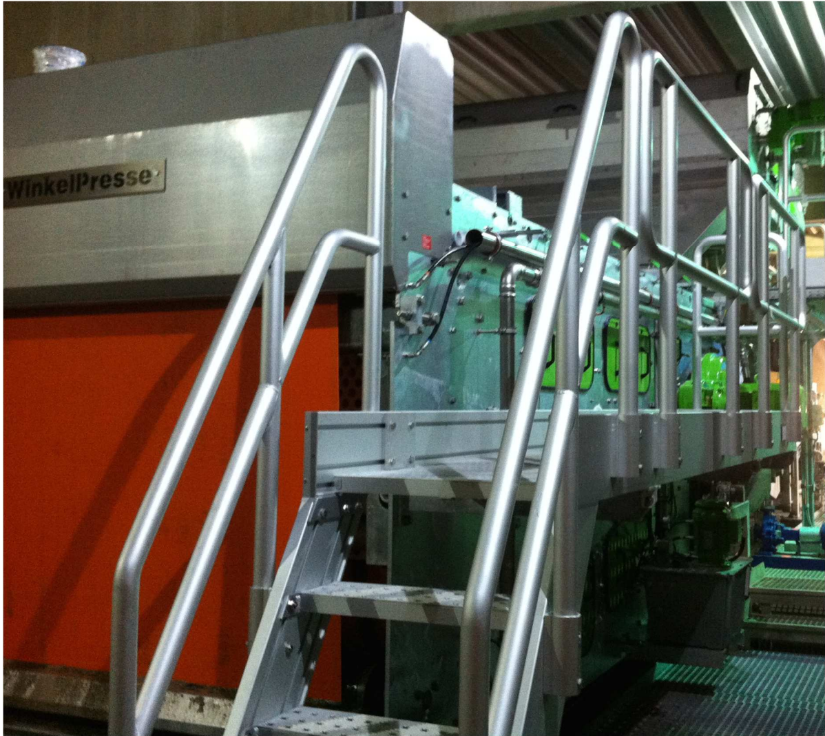
Figure 18: pre-thickener and high pressure belt filter press
